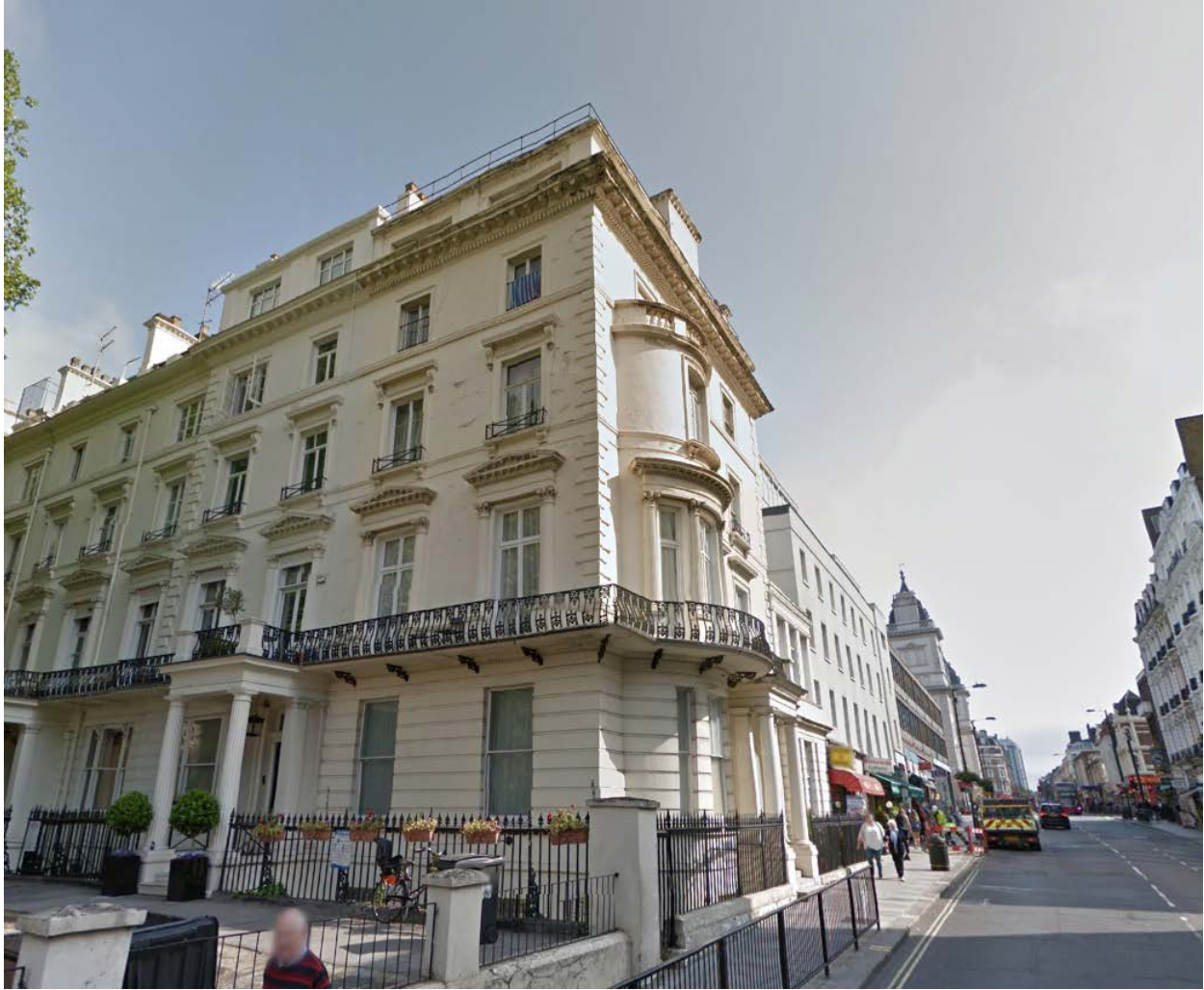
View of building from Westbourne Terrace.
